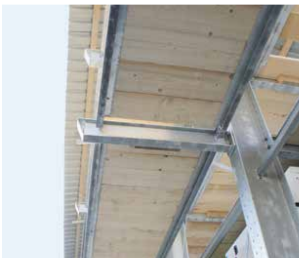
1 Underbridge beam on cantilever beams
